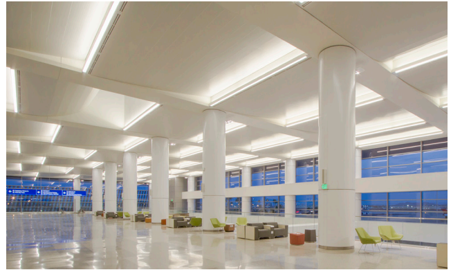
Project: PHX Sky Harbor - Terminal 3, Phoenix, AZ; Segmented Torsion Spring Photo Credit: Ed Taube
